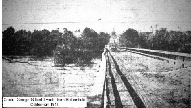
Jewett Lane Bridge (view south, 1911)
